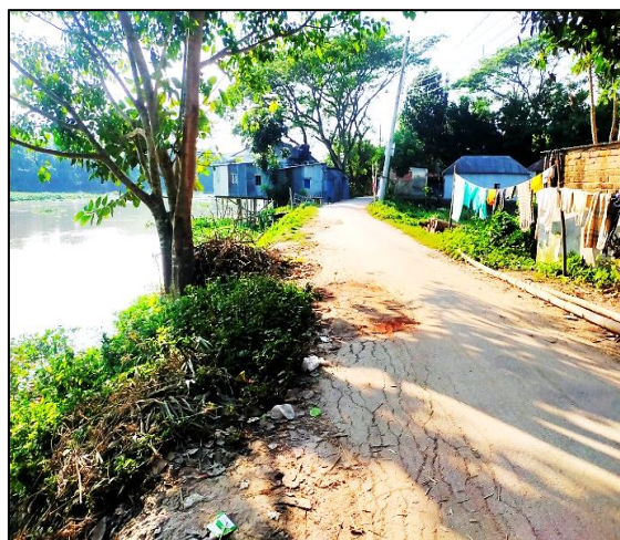
Road-01, Bhanga Paurashava
